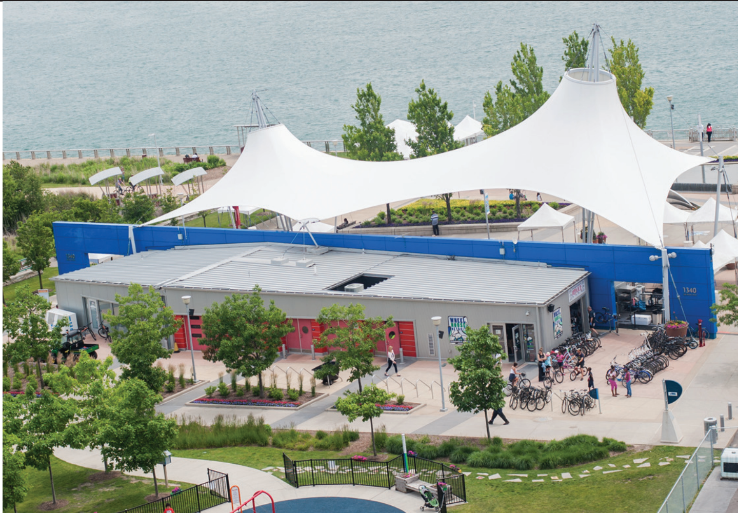
Not your image of Detroit, is it? Rivard Plaza, on the Detroit River, is home to Wheelhouse Detroit, the 500 square feet of the building where all the action is.
